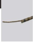
Use the wire strippers to carefully remove approximately 40mm of the outer sheath to expose the earth braid which surrounds the heating cores.
